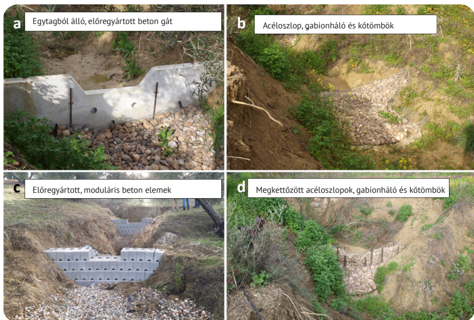
Fig. 1: Control gully dikes with different construction techniques.
