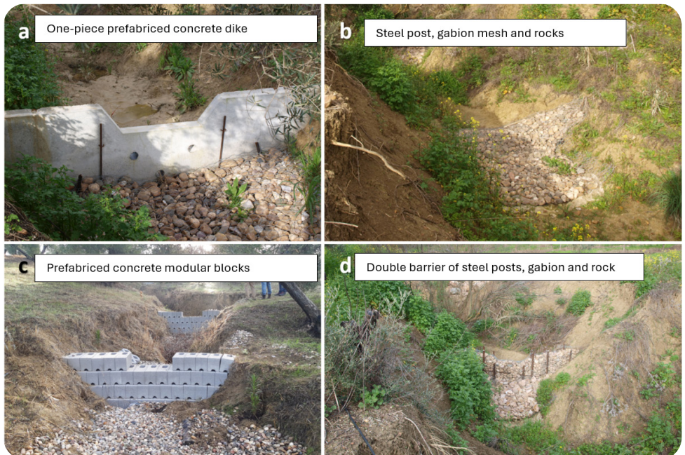
Fig. 1: Control gully dikes with different construction techniques.
